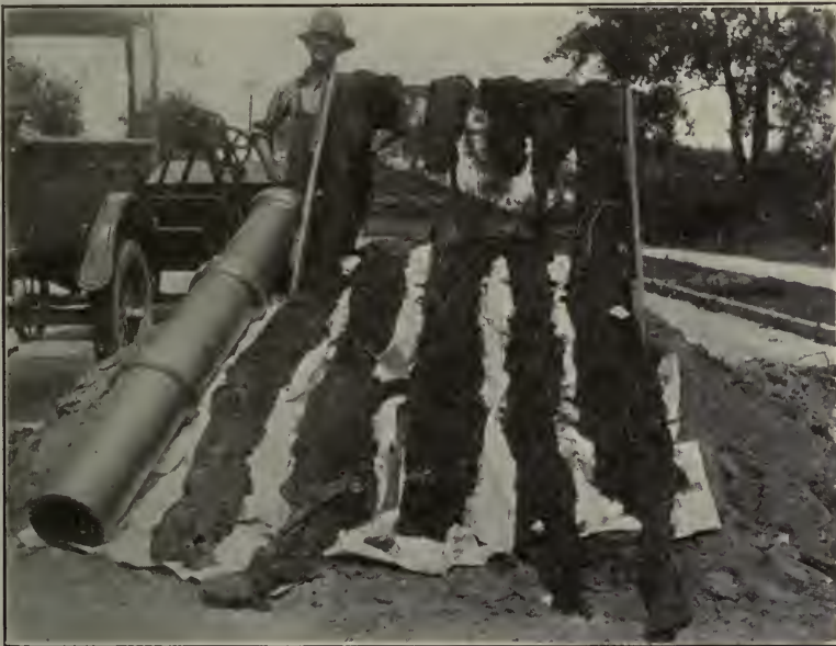
THIS ARRAY OF ROOTS FROM 100 FEET OF SANITARY SEWER ON LINDEN STREET, SCHENECTADY, QUITE EFFECTIVELY HELD UP THE FLOW OF SEWAGE
